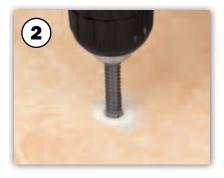
Once the hole has started, raise gradually the drill up to the vertical line.
